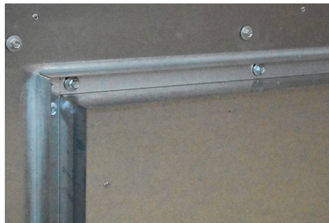
Double-Flange Duct Connection
