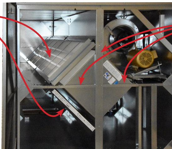
End View of Core Support Assembly
