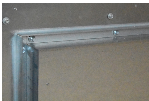
Double-Flange Duct Connection
