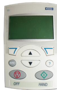
VFD Keypads Found in E-Box
