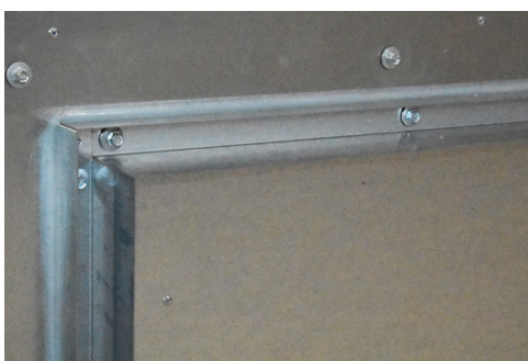
Double-Flange Duct Connection
