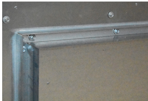
Double-Flange Duct Connection
