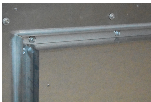
Double-Flange Duct Connection
