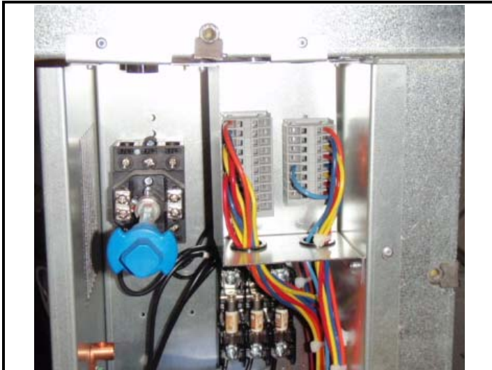
FIGURE 4-5 TERMINAL BLOCKS FOR CONTROL DEVICE CONNECTION.
