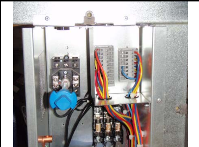
FIGURE 4-11 TERMINAL BLOCKS FOR CONTROL DEVICE CONNECTION.
