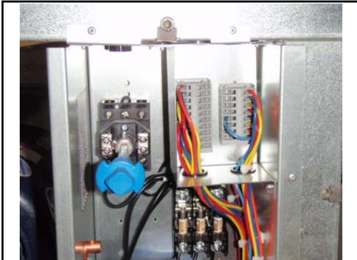
FIGURE 4-11 TERMINAL BLOCKS FOR CONTROL DEVICE CONNECTION.
