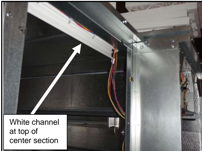
FIGURE 4-8 ROUTE CONTROL WIRES TO LOW-VOLTAGE E-BOX
