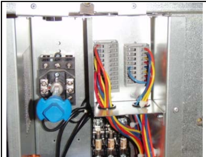
FIGURE 4-11 TERMINAL BLOCKS FOR CONTROL DEVICE CONNECTION.
