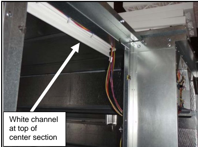
FIGURE 4-8 ROUTE CONTROL WIRES TO LOW-VOLTAGE E-BOX
