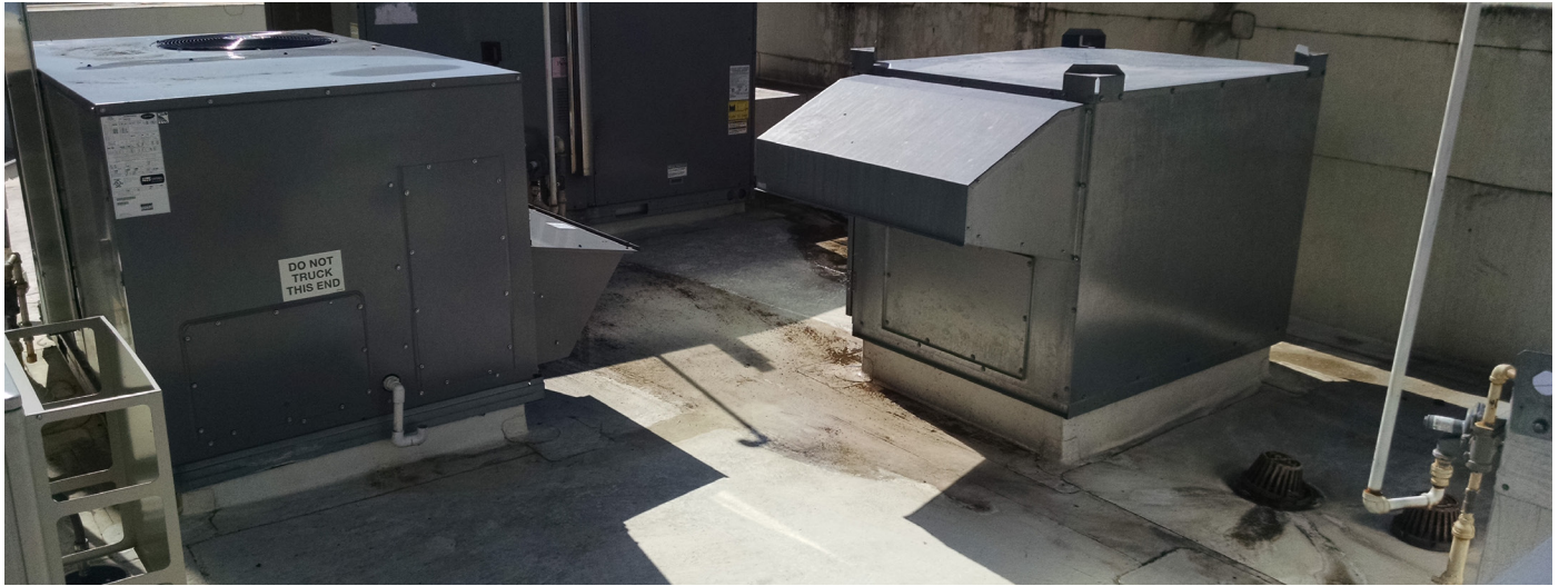
Rooftop units of the Hilton Garden Inn's HVAC system Image courtesy of Steve Coppock, Habegger Corporation
