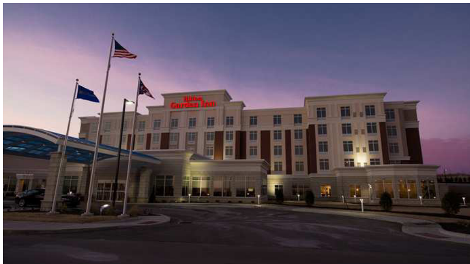
RenewAire ERVs reduced the annual HVAC energy use by 34% at the Hilton Garden Inn located in Dayton South/Austin Landing, Ohio
