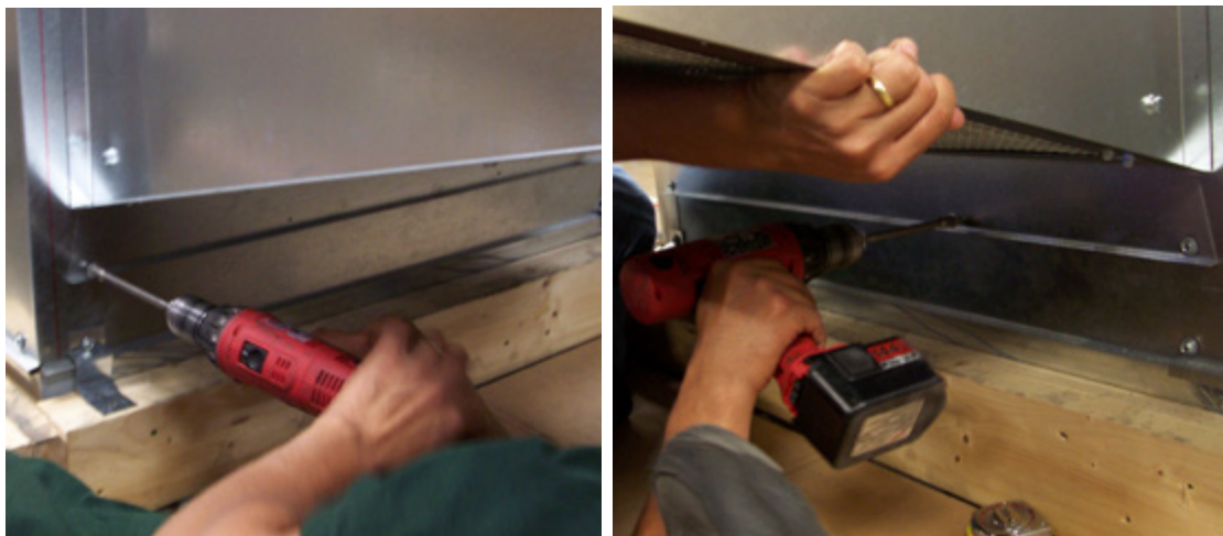
FIGURE 1.2.4 INSTALLING PLATE
