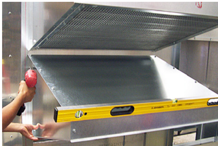
FIGURE 1.2.2 INSTALLING MIDDLE HOOD
