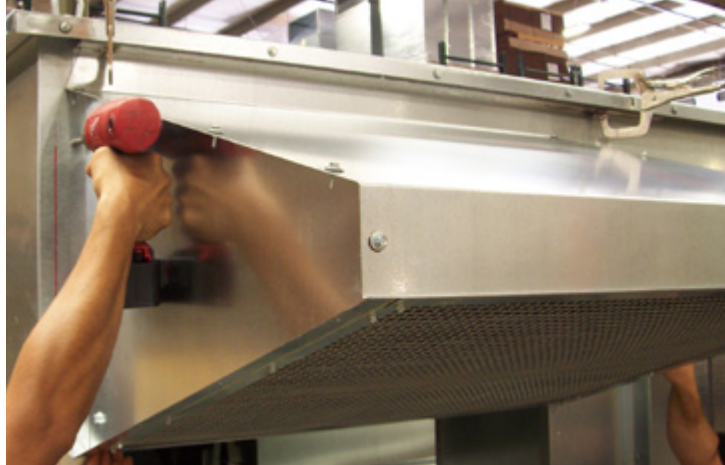
FIGURE 1.2.0 INSTALLING TOP HOOD
