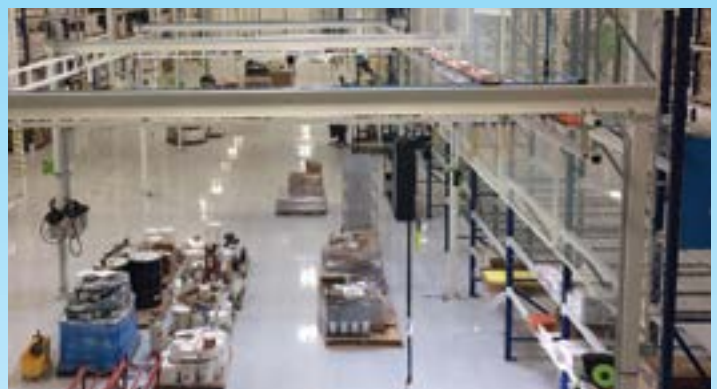
The new facility is more than double the size of the previous one and offers high indoor air quality
