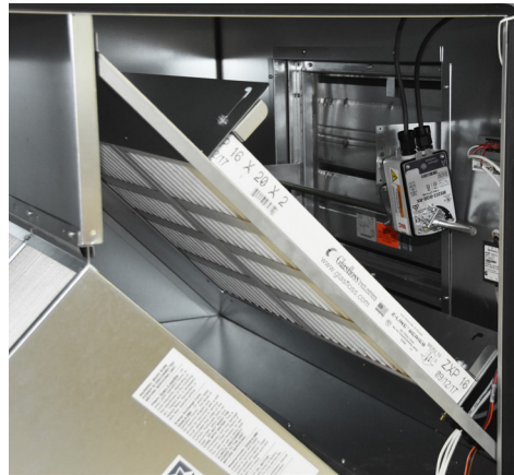
FIGURE 2.3.1 OA DAMPER AND ACTUATOR
