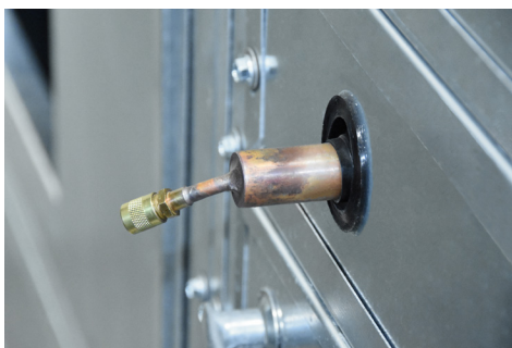
FIGURE 5.5.0 SUCTION LINE FOR DX COIL
