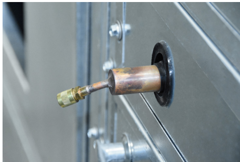
FIGURE 5.7.0 SUCTION LINE FOR DX COIL
