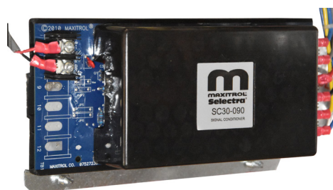
MODEL SC-30 USED TO ACHIEVE 10:1 TURNDOWN IN 3-VALVE SCHEMES MODEL SC-40 USED TO ACHIEVE 5:1 TURNDOWN IN 2-VALVE SCHEMES
