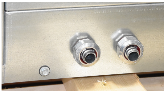
FIGURE 7.10.0 ELECTRIC SUPPLY FITTINGS (TYPICAL)
